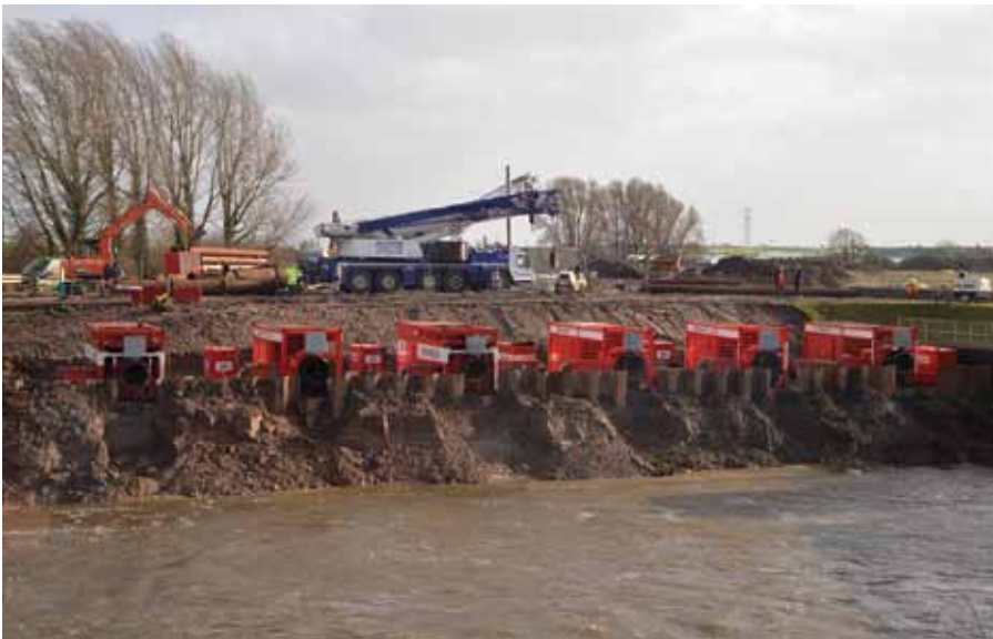
The scale of the Dutch pumps used for emergency flood water removal in 2014 on the Somerset Levels.
